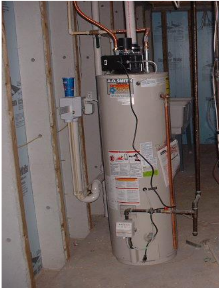
Power Vented Water Heater
