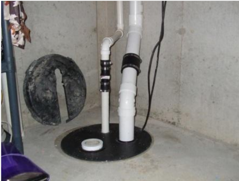
Sealed Sump Pump
