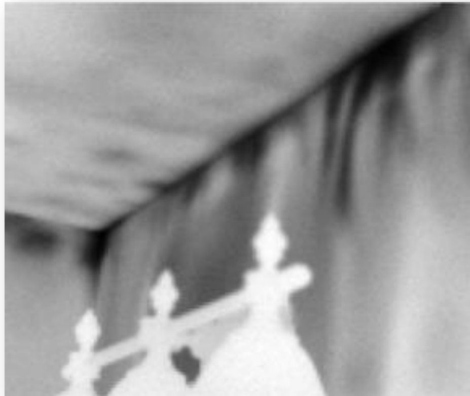
Attic air infiltration into the wall
