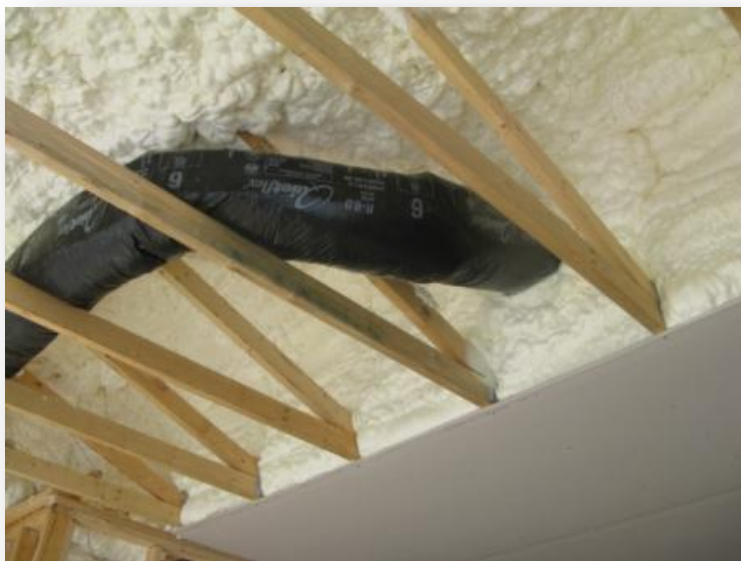
Ducts in unvented attic
