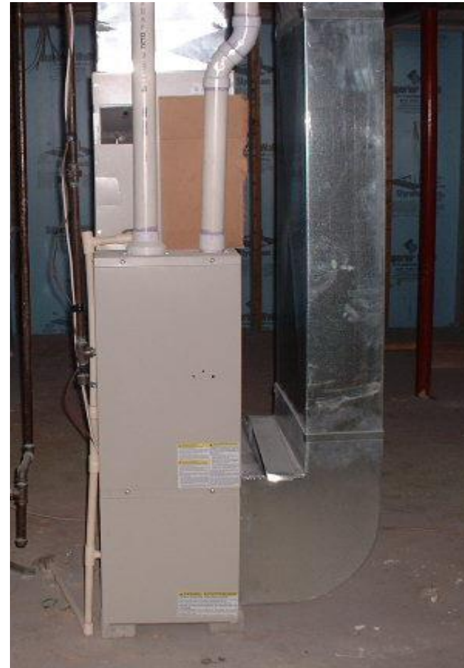
Direct-Vent Furnace
